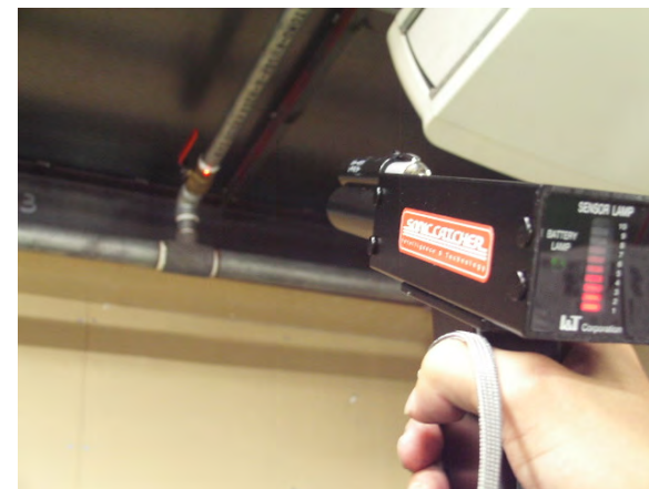
Air leak test
