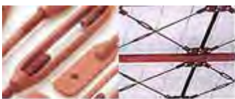
JIS brace for quake-resistant structure
