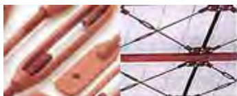
JIS brace for quake-resistant structure
